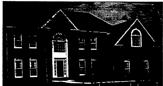
Multiple Hip and Gable Roofs Combined
