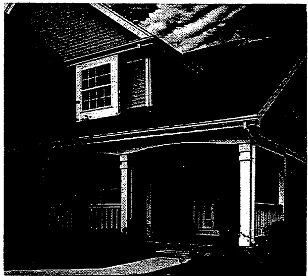
Porch Entry & Second Floor Bay Projection
