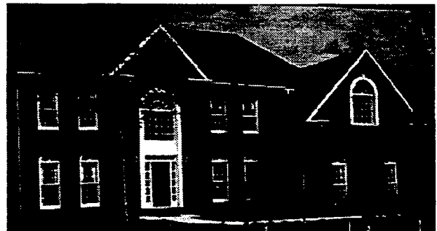
Multiple Hip and Gable Roofs Combined
